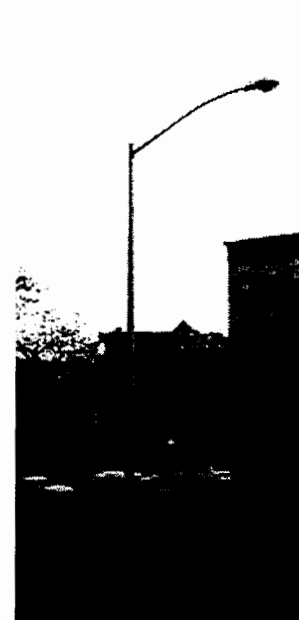
cobra head fixture
