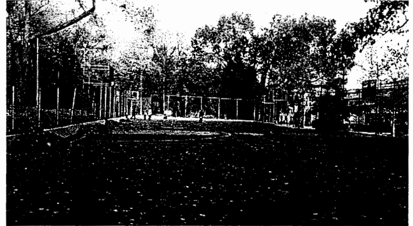
existing courts to be repaired
