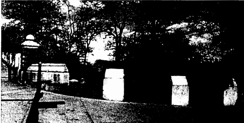
existing park entry at Morningside Drive and 110 th Street
